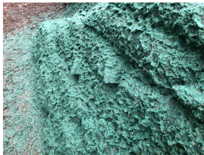
Freshly hydroseeded bagwork
