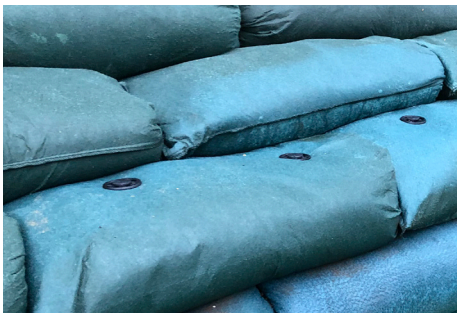
Newly placed bagwork
