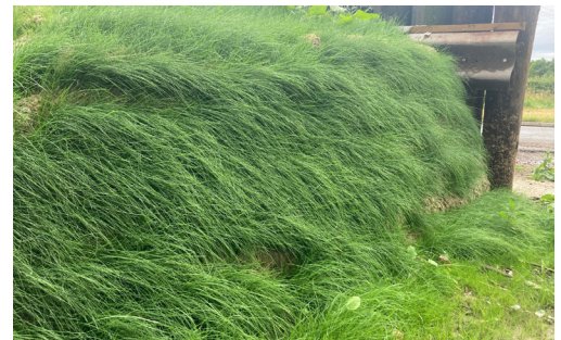
Hydroseeded bagwork after 8 weeks
